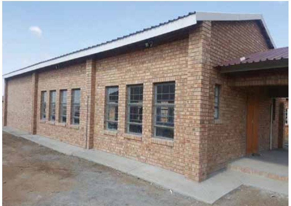
New school hall built in Mpumalanga
