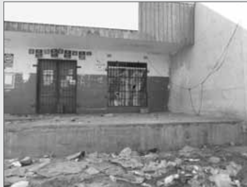
Figure 2: Examples of the damage caused to businesses as a result of xenophobic attacks; where the business owners had Sasria cover and could be reimbursed for their losses
