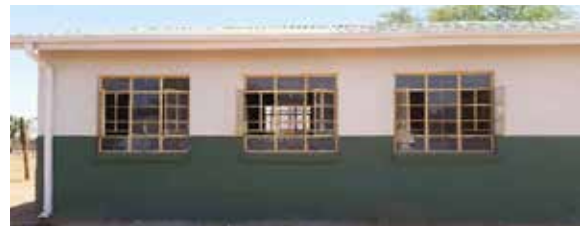
Merwe High School in Limpopo before and after the renovations
