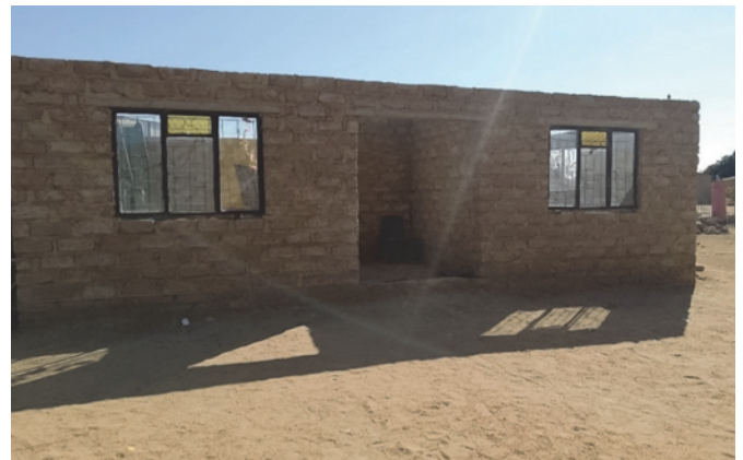
Mandela Day project before the renovations
